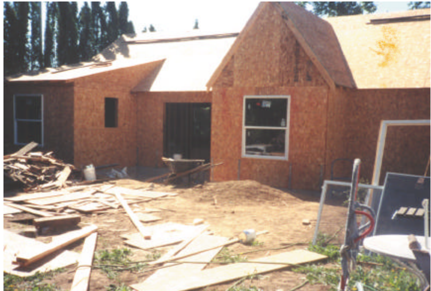
Sheathing is done. View from the new backyard.
