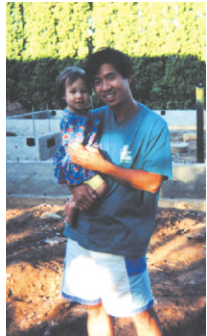
Luke takes a break from building the foundation of the rental house to show it off to his daughter Abriel.
