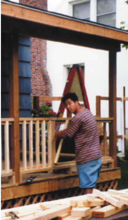
Building a covered deck behind my house
